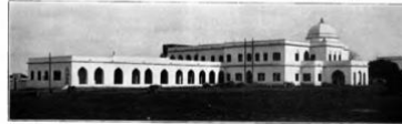
View of Hospital, about April, 1928, before completion. Main Ward to left, Central Block, entrance, Completed Dispensary, Operating Room, Examination Rooms, X-Ray and Vaccination Department.
